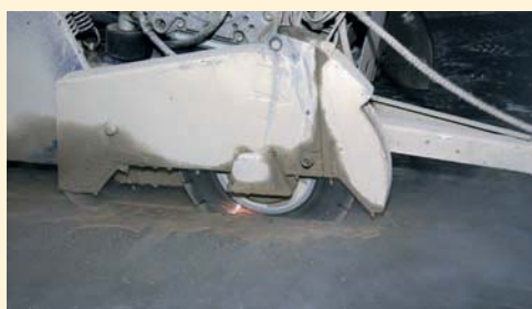
>>> Sciage des joints.
